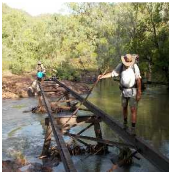
Crossing the old bridge over Koolpin Creek
