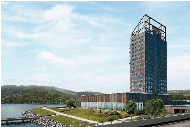
The Mjøsa Tower in Brumunddal, Norway, will be the world’s tallest wooden building
