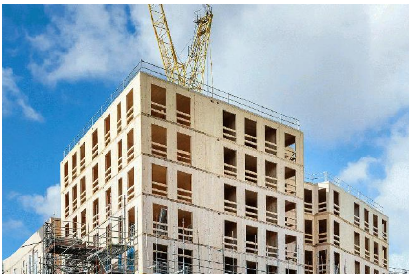
Mid-rise wooden buildings, like these in London (above and below), can be put together in a few days
