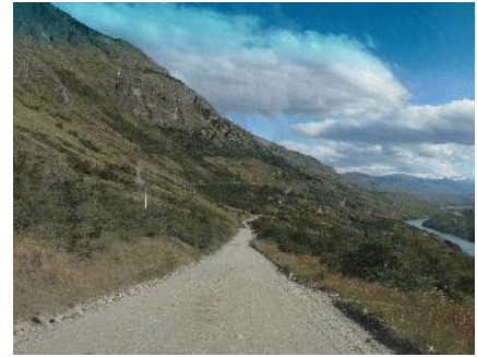
Looking down the Carretera Austral, the main 'highway' in southern Chile
